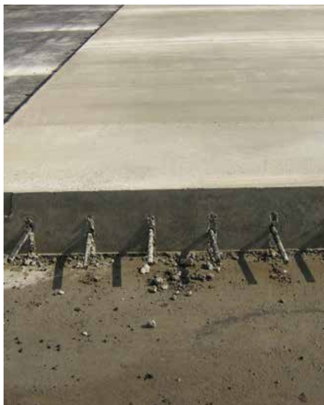
Joint de construction transversal
