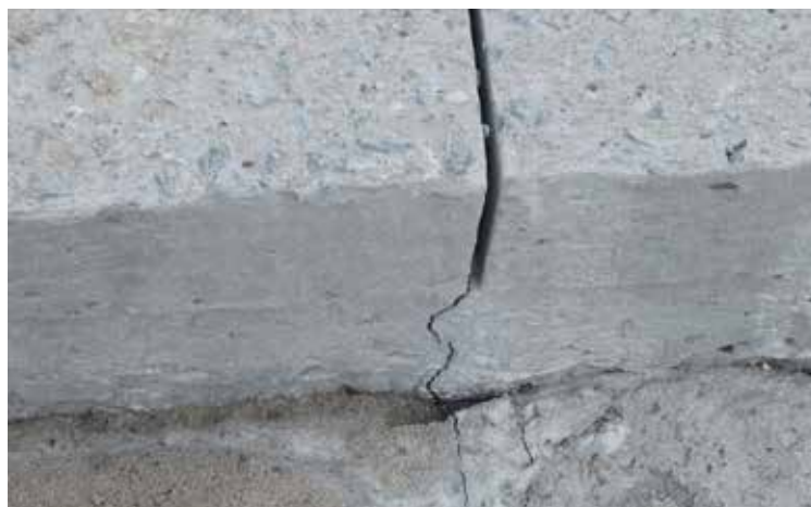
Sciage servant d'amorce de fissuration
