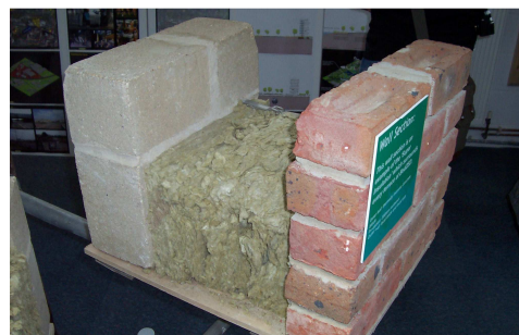
Figure 2d: Section through a very highly insulated external wall with a heavyweight concrete inner leaf for good thermal mass. This provides excellent year-round thermal performance by creating an optimised combination of energy flow and storage. (Photo taken during study tour at BedZED, UK)
