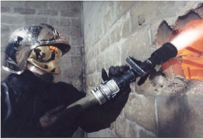
Breach in a fire wall (source CIMBETON)
