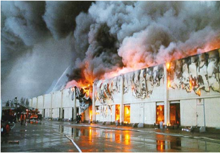
Figure: Cell of 5000 m 2 - Heat flux without fire wall (source CIMBETON).
