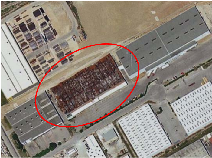
Figure : 7200 m 2 industrial warehouse North Rognac (France) - Saturday 15 th June 1996 (source CIMBETON) : The concrete fire walls isolated the fire perfectly and prevented it from spreading to adjacent warehouses.
