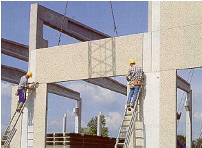
Concrete curtain walls with CF 2hr heat shield (source: CIMBETON)
