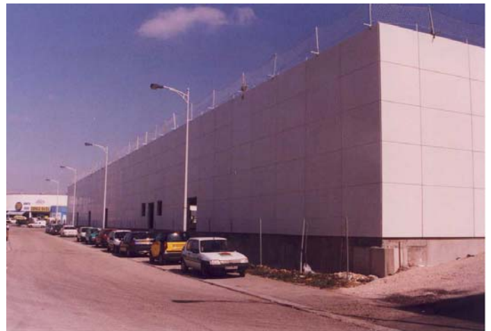
Fire-retardant façades (source: CIMBETON)
