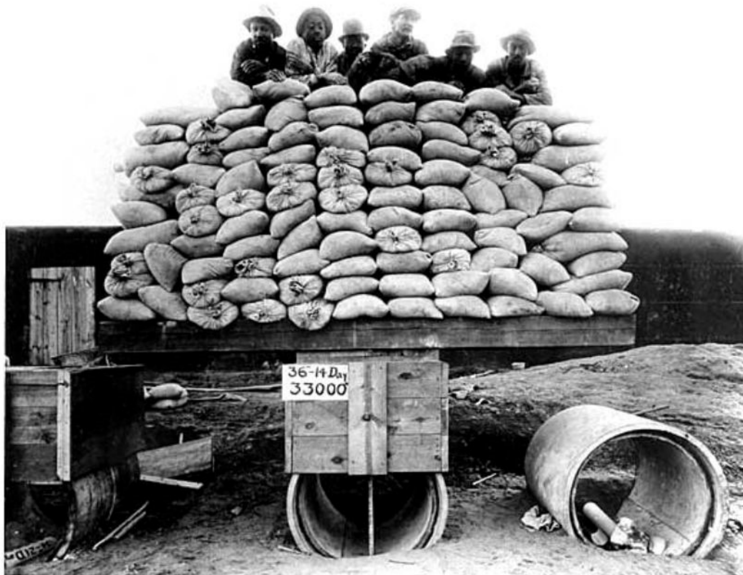
Load test on Concrete Pipe 1914 City Archives of Philadelphia
