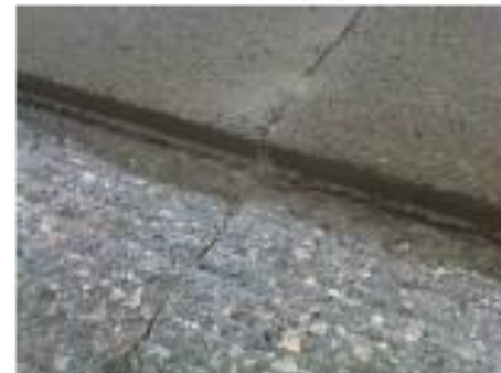
Thin concrete overlay
