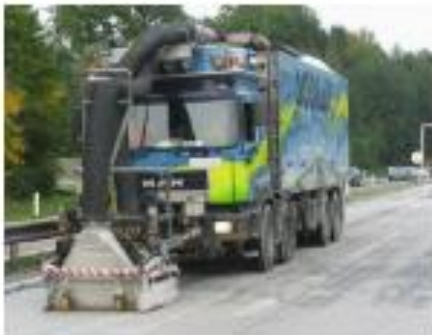
Milling of the old concrete
