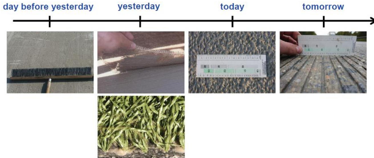
Image 2: Development of the standard concrete surface on German trunk roads (from left to right: steel broom, burlap cloth and artificial turf, exposed aggregate concrete, grinding with grooving)
