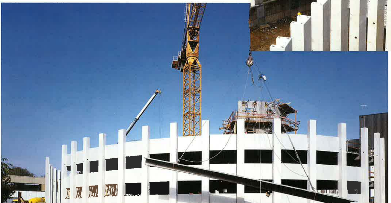
Smithkline Beecham, Rixensart - SAMYN and PARTNERS, architects and engineers (photos M. Detiffe)
