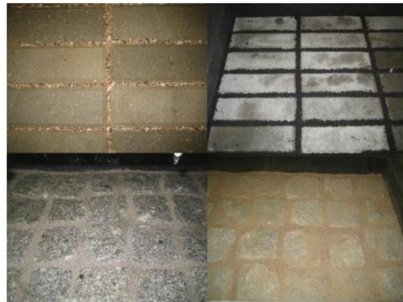
Figure 2. Concrete blocks with 1/5 sand joints (top left) and composite joints (top right). Natural stone with composite joints (bottom left) and 0/4 sand joints (bottom right).
