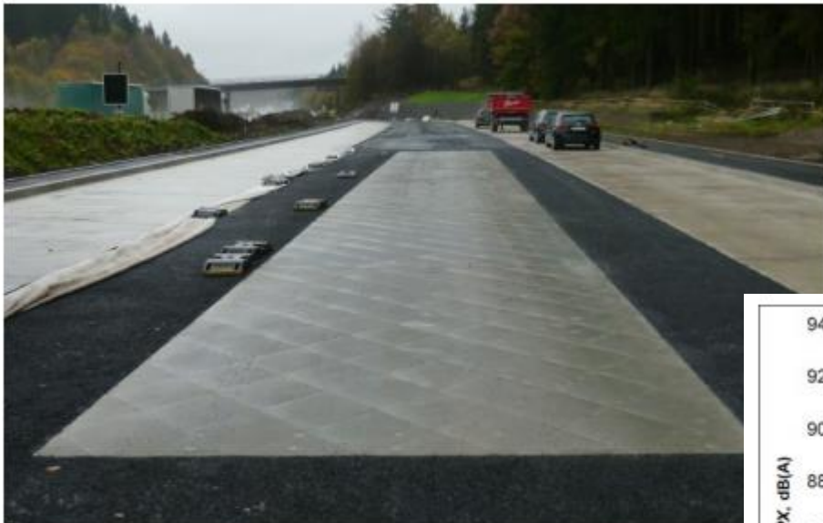
Figure 4. UHPC test track after completion?
