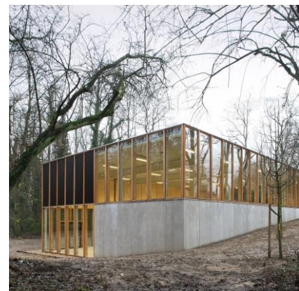
Bureau arch. URA – © photo Filip Dujardin
